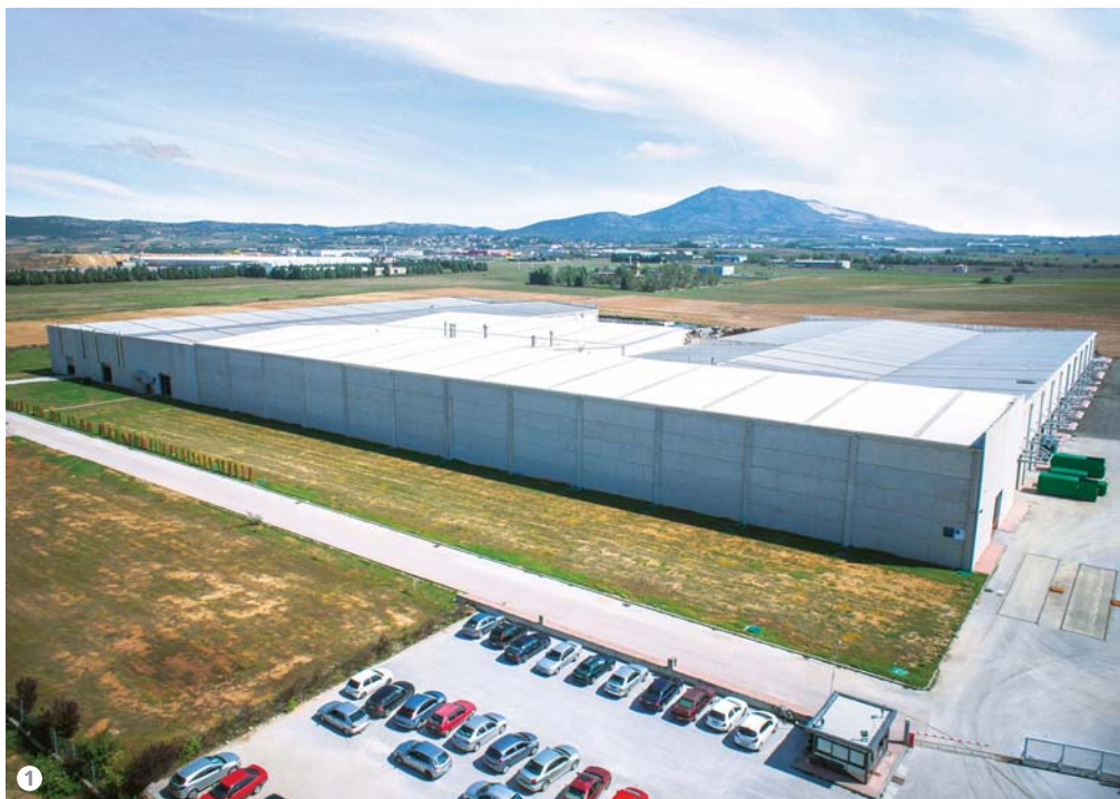
Figure 1: The new production site of ELVIAL, built in 2005 in Kilkis (Greece).
